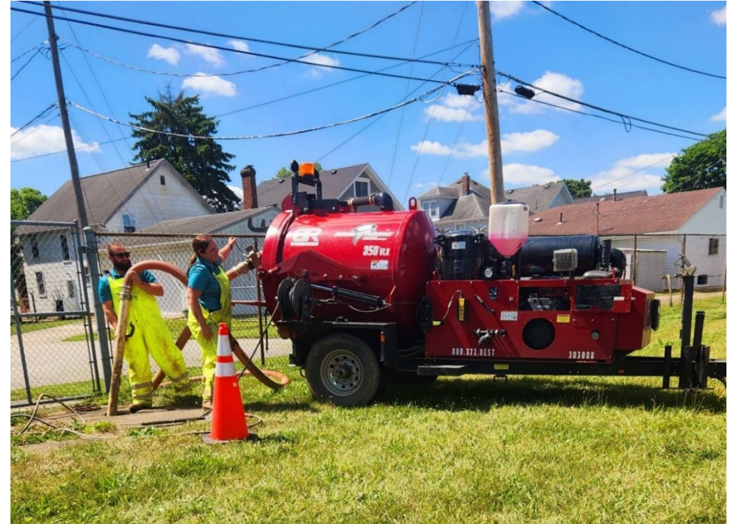
Service-Line Verification Pot-Holing Demonstration RCAP Field Day, 06-11-2024
